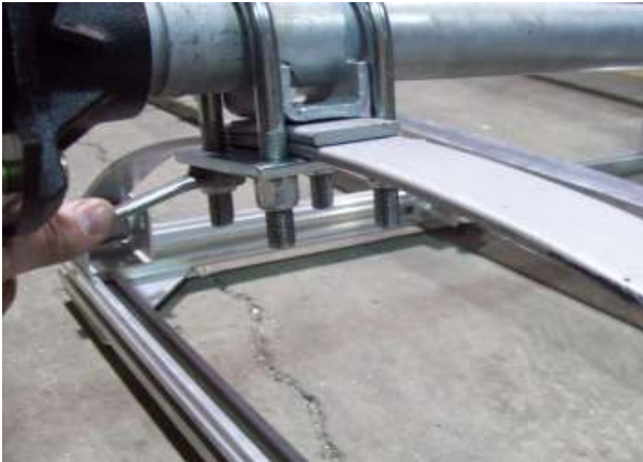
Install the U-bolts and tie plates and nuts. Tighten nuts evenly as shown.
